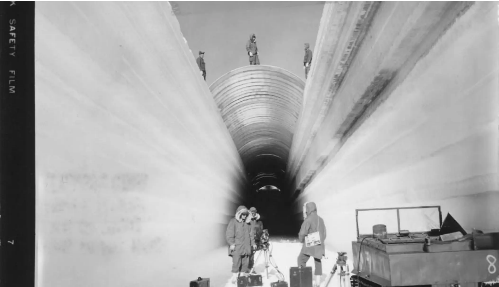
Camp Century construction under way, building tunnels into the ice. (Photo: US Army)
